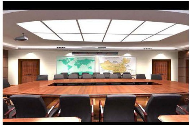
Embedded LED Panels in China
