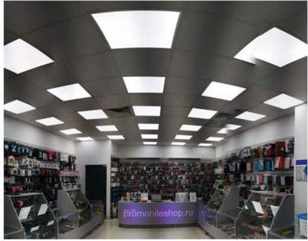
Embedded LED Panels in Russia
