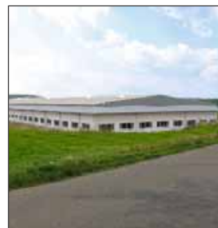
6. Markersdorf / Saxony Production of the buckles
