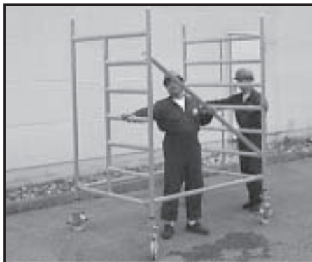
Figur 11 Diagonalstiver monteres
