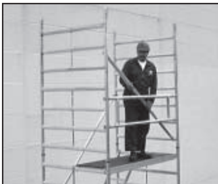
Figur 21 Diagonalstiver monteres
