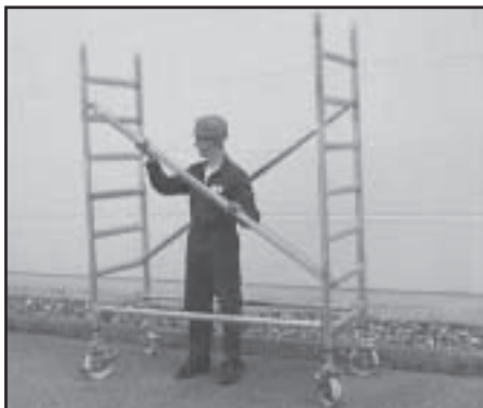
Figur 16 Diagonalstiver monteres
